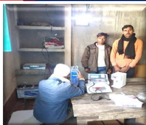
Dairy MCC – Village Bhullo
