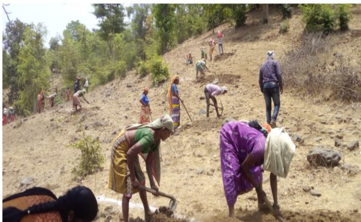
Farmer beneficiaries digging Continuous Trenches (CCT) in Mokhada, Palghar
